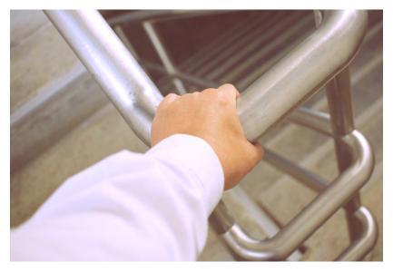
There are also specific rules and regulations around guardrails. Top rails should be between 39 and 45 inches from the walking surface, and openings should not exceed 19 inches wide. Rails must also be able to resist 200 pounds to the top rail and 150 pounds elsewhere - without fail. Guardrails are the most basic way to prevent falls to lower levels, which claimed 697 worker lives in 2016, according to the BLS.
